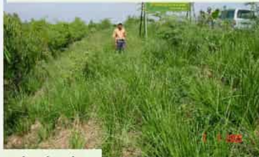
Effectiveness of vetiver planting in protecting dikes from flood erosion
